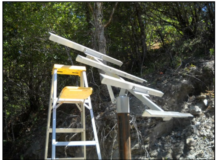
Pole Top Mount on a six inch steel pole. The pole is set in concrete.
