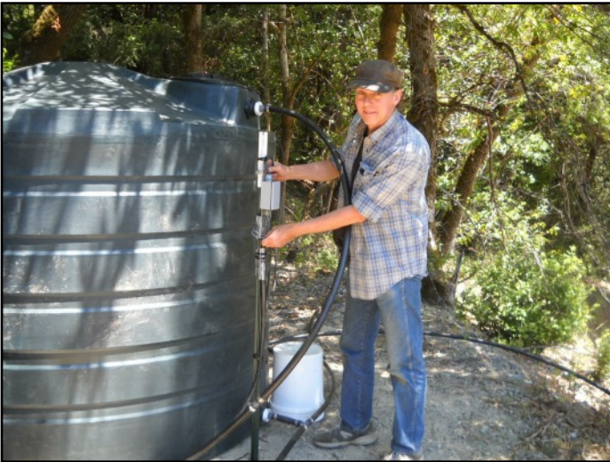
Making the float switch connections.
