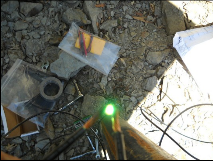
These solar panels are so powerful when they are wired for 48 volts, that they are capable of striking an arc if the cable ends touch, so be careful.
