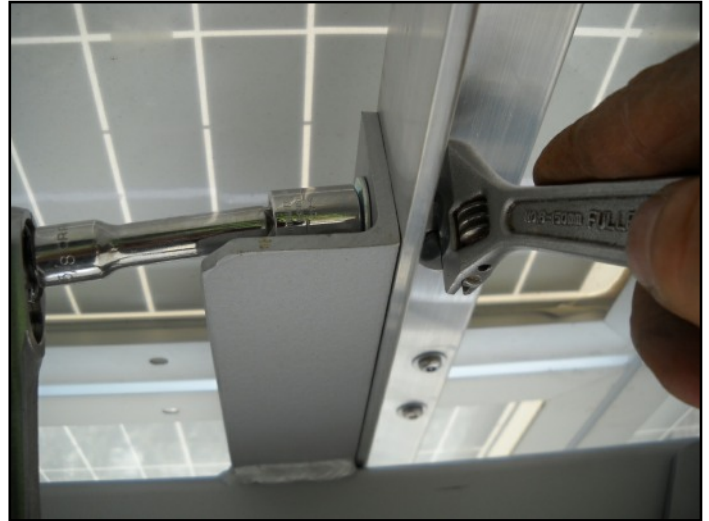
Leave the ribs loose on the strongback until you have all the panels installed, because you may have to move the panels around a little to get everything to line up.
