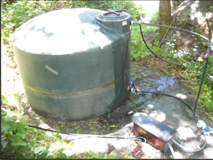
Feed tank and pump
