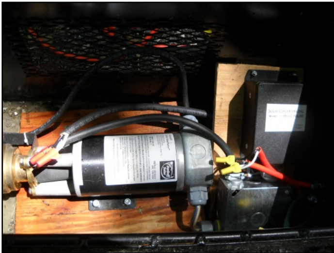
Dankoff pump and pump controller mounted on a board and installed in the lockbox.
