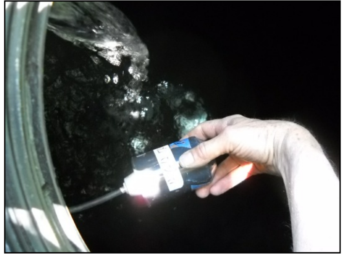
Float switch in the receiving tank stops the pump when the tank is full. It is connected to the pump by 150 feet of 18 gauge, two conductor cable. We used a fish tape to run it inside of 1/2" poly pipe for protection. The same with the array to pump cable, it's also inside poly pipe.
