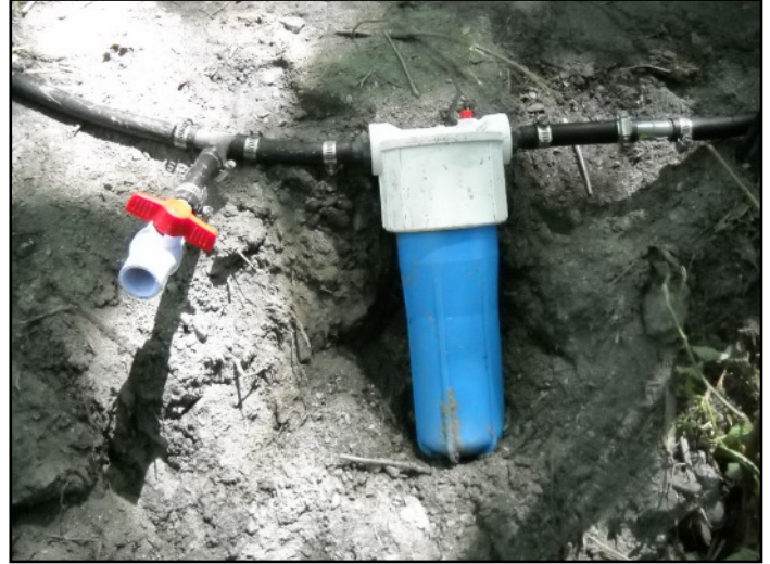
10 micron filter assembly, a necessity for these pumps.
