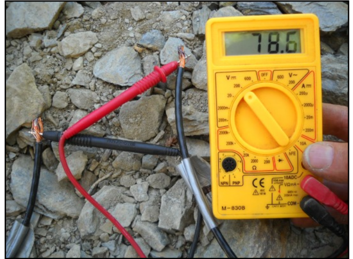
Four 12 volt panels were wired in series. Theoretically that adds up to 48 volts but with no electrical load on the panels, the voltage is much higher. When the pump is running, the voltage drops down considerably.
