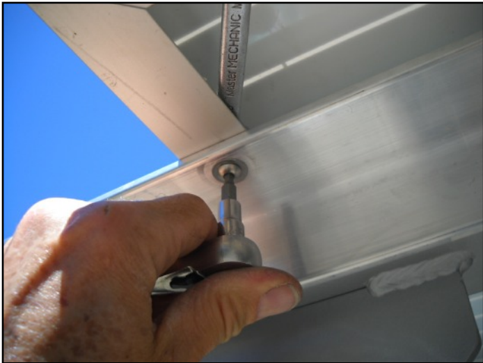
Using a 7/16" wrench and the Torx bit.
