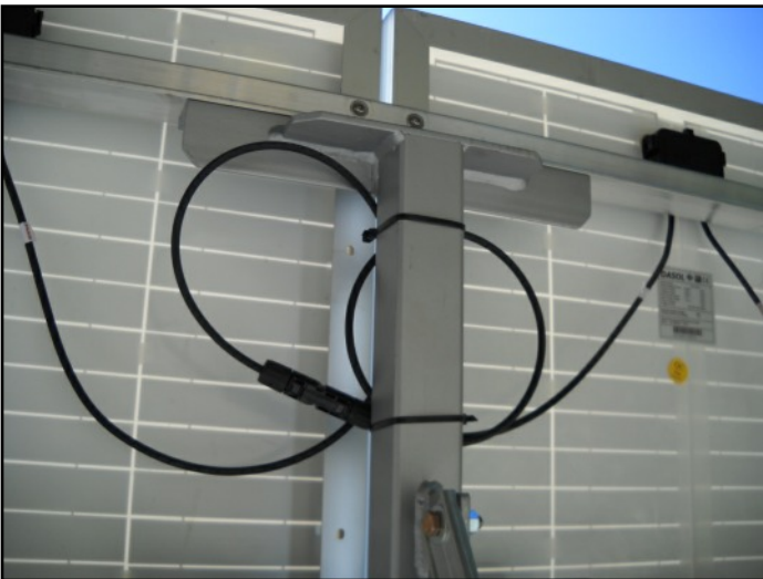
Coil up the cables and secure them with zip ties.
