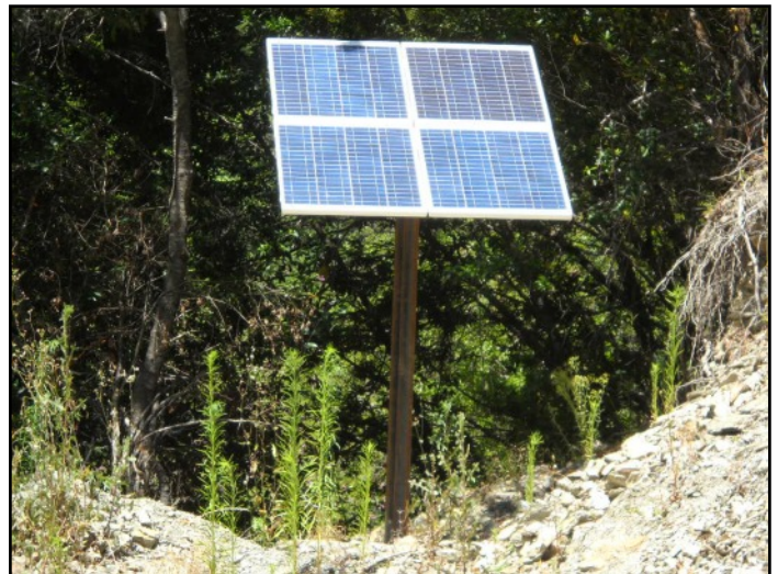
Four 60 watt, 12 volt solar panels were used.
