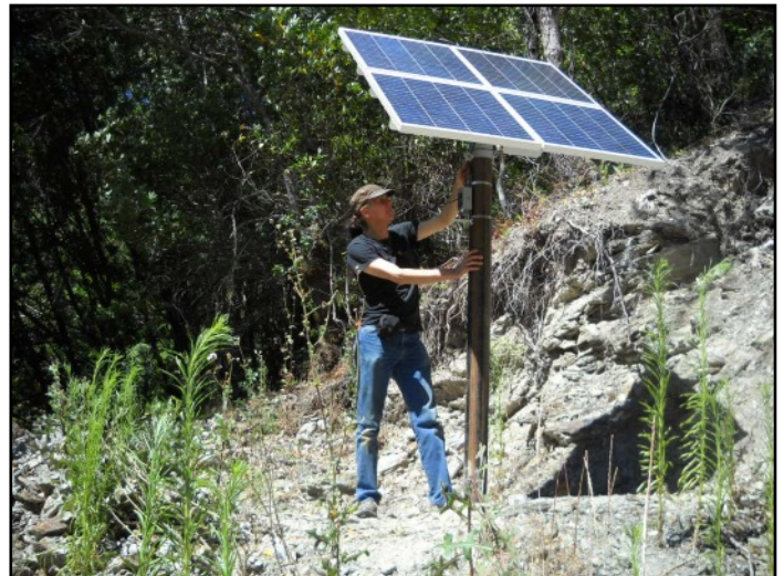
Yours truly Thad Horner putting the finishing touches on the panel installation.
