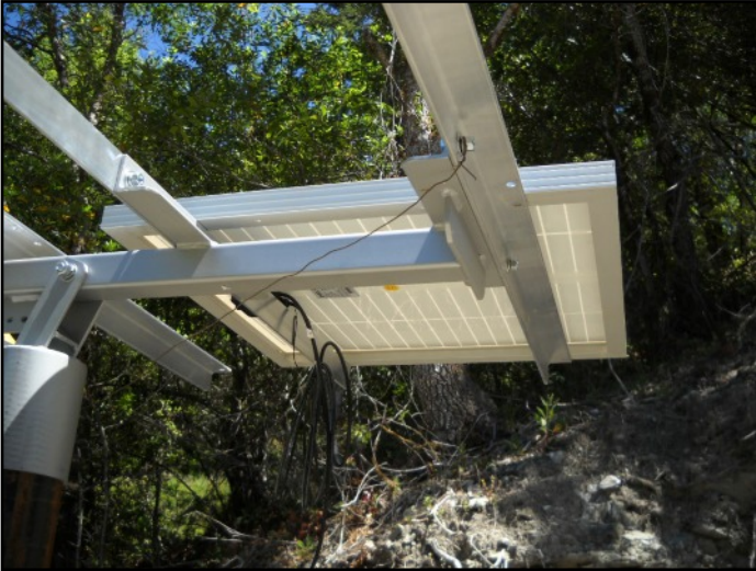
You can tie wire onto the frame to keep it from moving. If the frame is flat, it's much easier to mount the panels.
