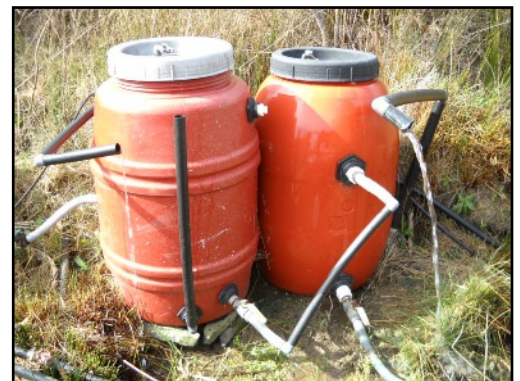
Double pickle barrel settling tank
