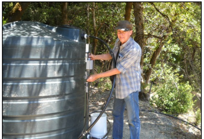
Putting the finishing touches on the wiring at the receiving tank. Pump will provide about 1,000 gallons per day.
