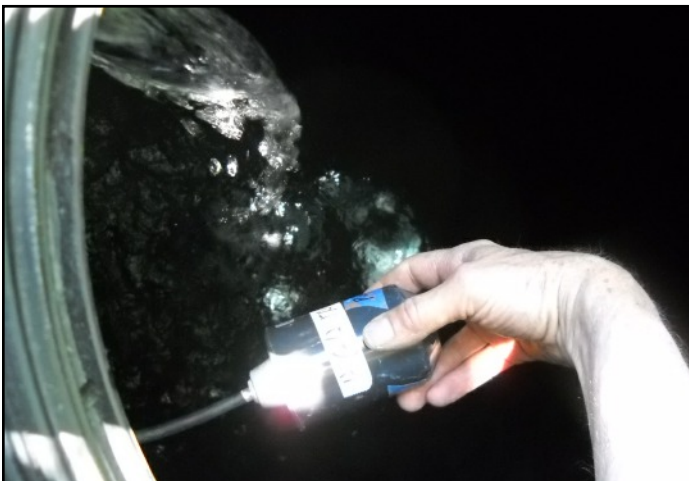
Water flows into the receiving tank. The pump is controlled by the float switch.
