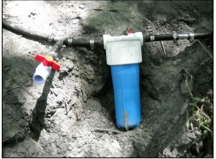
10 micron filter assembly for the pump
