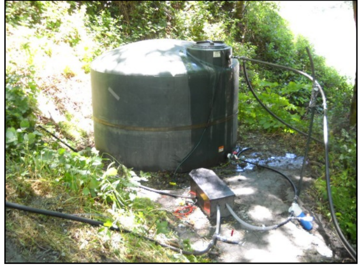
Storage tank receives water from the spring. Pump is in a waterproof, theft resistant lockbox.
