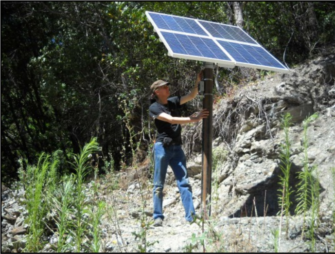
Solar array with four 60 watt solar panels is installed on a mounting pole and rack
