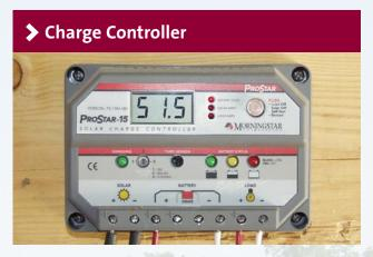
Morning Star PS15M-48V Charge Controller includes connections for solar input, battery output, and load output to the CU 200 and SQFlex
