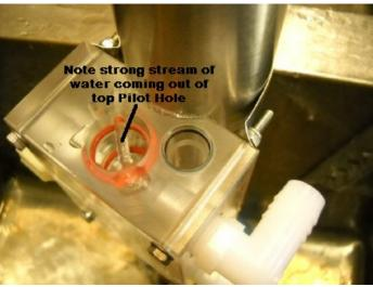
You can unclog the Pilot Holes with a tool shaped as below. You can make this out of a piece of wire taped to a stick. Find the three Pilot Holes inside the Barrel and insert the tool into them to push out the dirt. Then flow more water into the Barrel and recheck.
